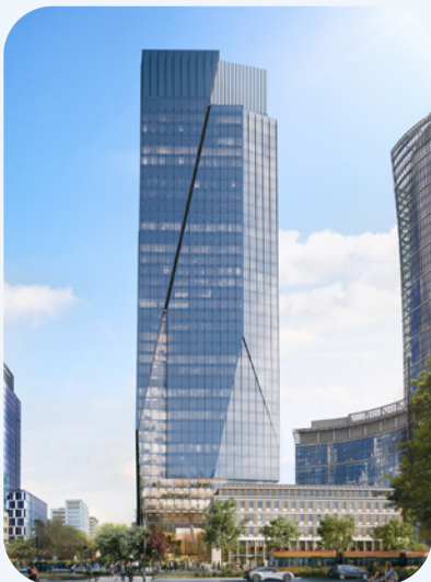
The Bridge is planned to have an operating system, which will allow for efficient access control management and solutions, increasing its safety.
