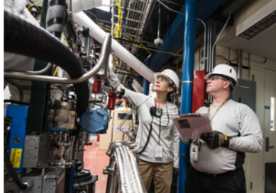
Alerting of the presence of moisture during production process
